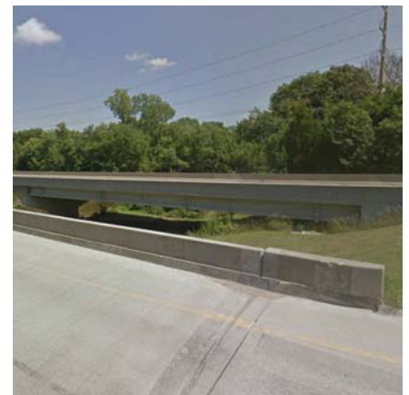
ROOM UNDER HIGHWAY 141 AT NW TOWNER DR.
