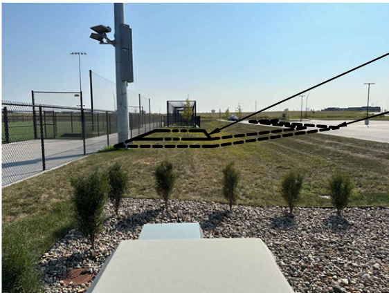
2 SITE PHOTO VIEW: LOOKING EAST
