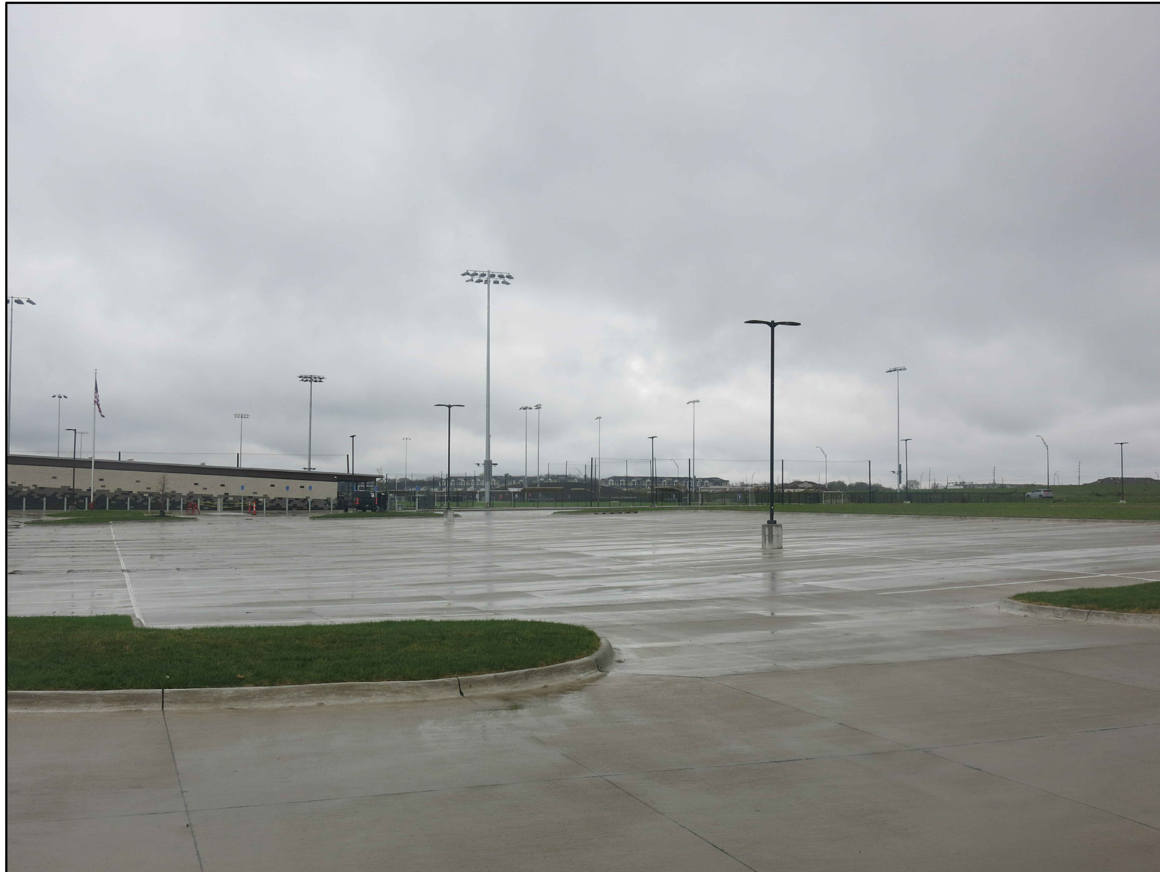
① EXISTING PHOTO
