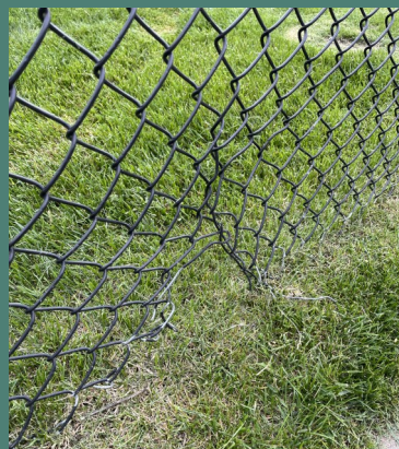
Existing Fence Damage
