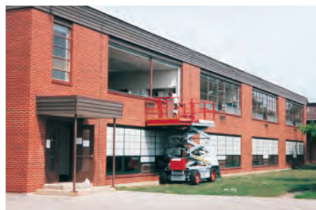
During Window Replacement
