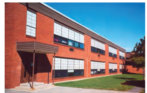
After Window Replacement
