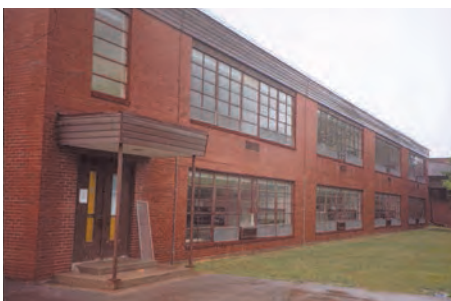
Before Window Replacement
