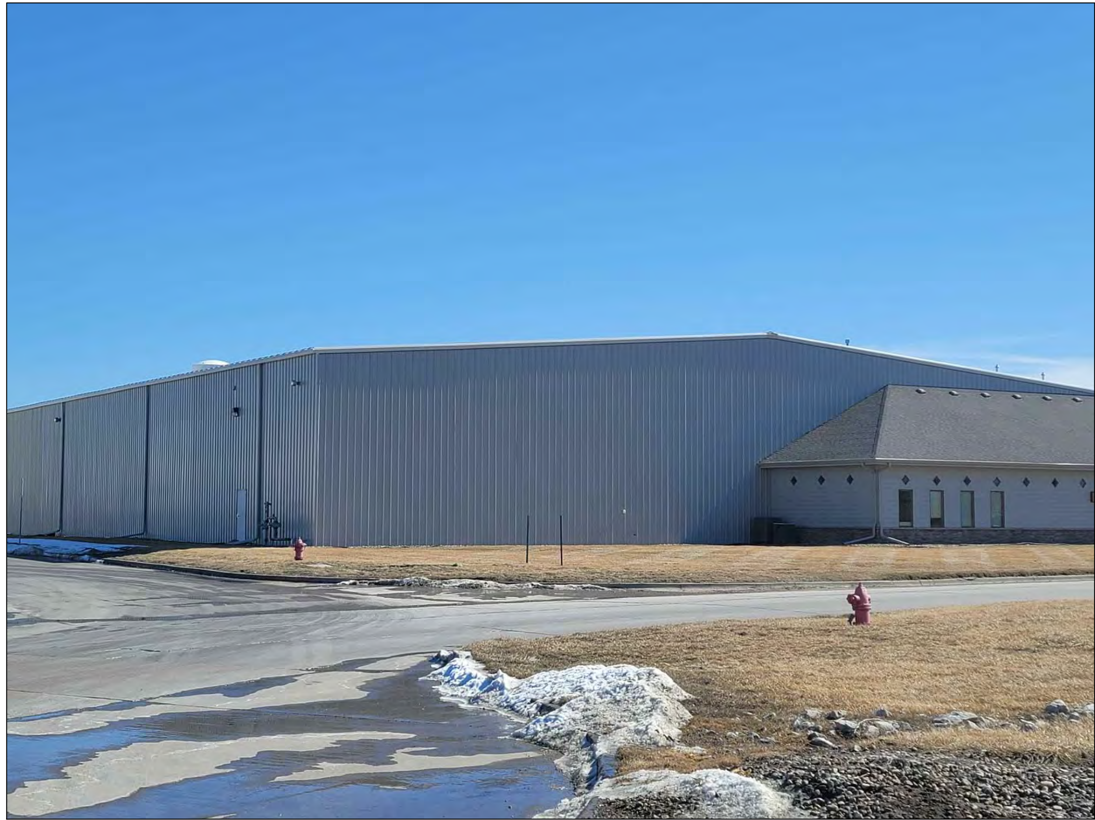
ADJACENT BEISSER BUILDING
