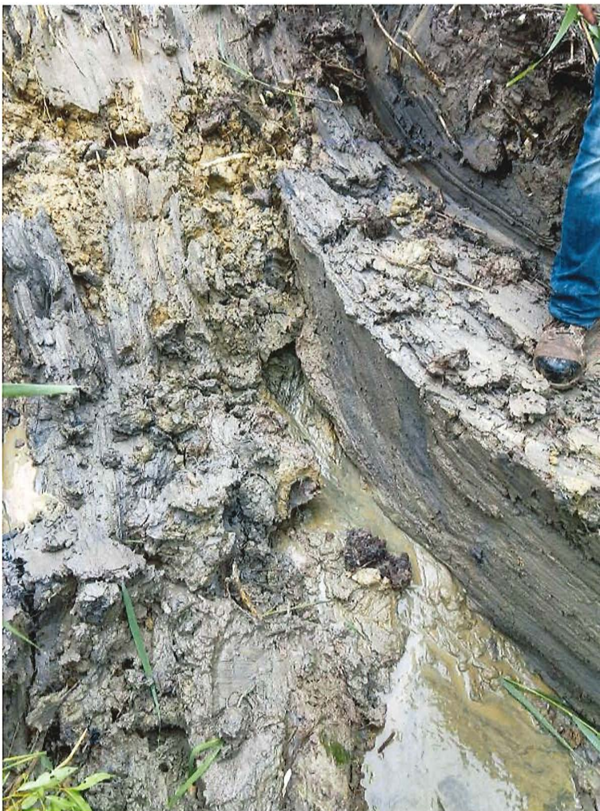
Photo No. 3 - Saturated Sand (flowing) - Test Pit Near Station 104+00
