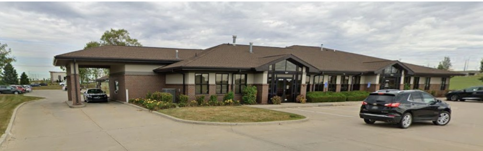
Existing Building with Drive-Thru
